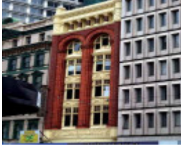
B4618 Paton Building
