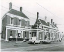
B5560 Court House & Police Station
