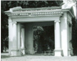
B0437 Greek Pavilion Fitzroy Gardens East Melbourne
