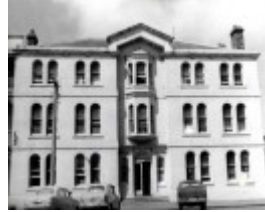
B0871 Mac s Hotel Gawler Street facade
