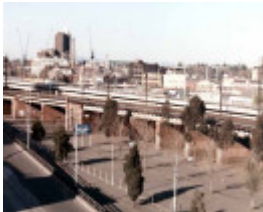
B5747 Flinders St Rail Viaduct
