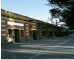
B5747 Railway Viaduct
