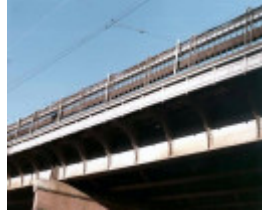
B5747 Flinders St Rail Viaduct
