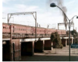
B5747 Flinders St Rail Viaduct
