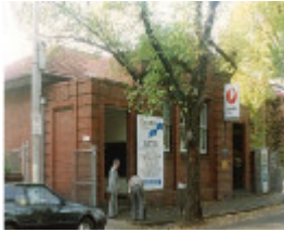
B6420 Former Post Office
