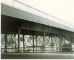
B1600 Metal Truss Bridge
