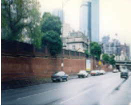
B6442 Retaining Wall
