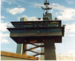
B7180 Shipping Control Tower
