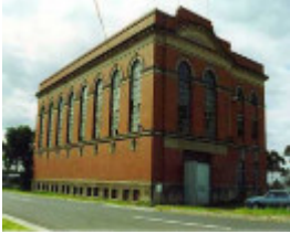
B3682 Albion Sub-Station
