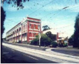
B6151 Tram Depot
