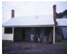
mt mitchell homestead & stables sunraysia hwy lexton stables outbuildings jul83
