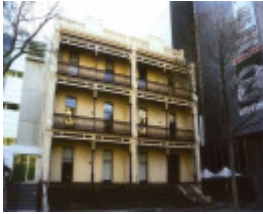
B6622 Former Lonsdale Private Hospital
