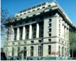
B4119 Fmr Port Authority Building
