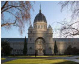
B0842 REB and Museum Victoria Verandah
