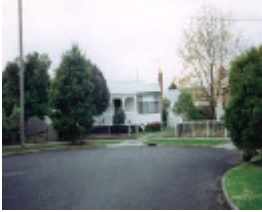
B6526 Railway Workers Cottages
