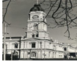
B2388 Town Hall North Melbourne
