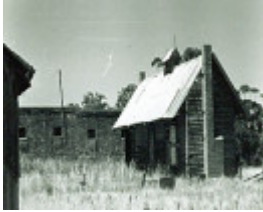
B3753 Police Stud Buildings
