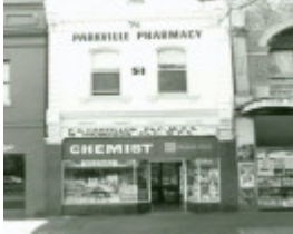
B4721 Frmr Parkville Pharmacy Facade
