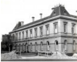
B0425 Police Offices
