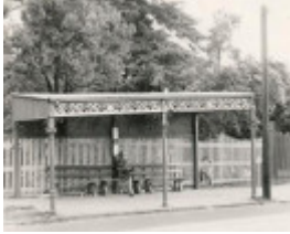
B3312 Cast Iron Tram Shelter
