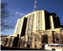
B6372 Former Police Headquarters
