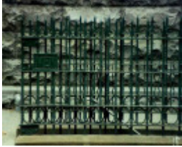
B6720 Underground Conveniences
