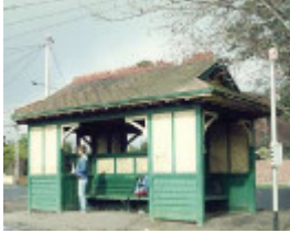
B7040 Tram Shelter
