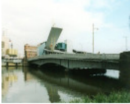
B6799 Spencer Street Bridge
