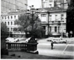
B0074 Former Campbell Residence
