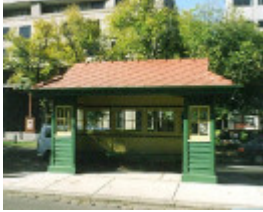
B7043 Tram Shelter
