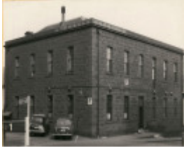
B1254 Victoria Barracks F Block
