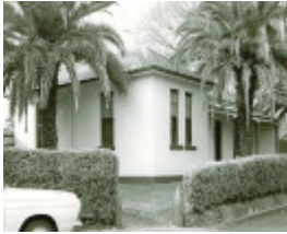
B3106 Victoria Barracks Caretakers Cottage
