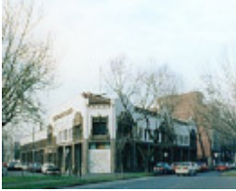
B4870 Former Car Showroom
