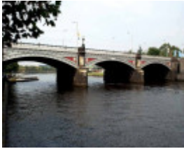
B2238 Princes Bridge
