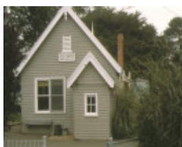
little hampton primary school no 1700 side view
