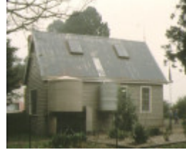
little hampton primary school no 1700 rear view
