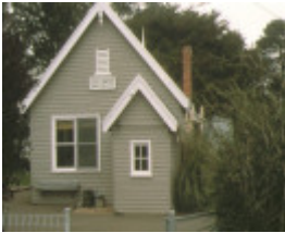
little hampton primary school no 1700 side view
