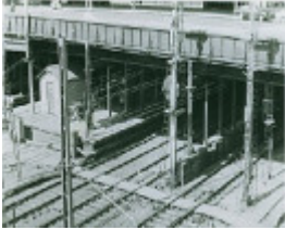
B3120 Swanston St Bridge Over Rail Lines
