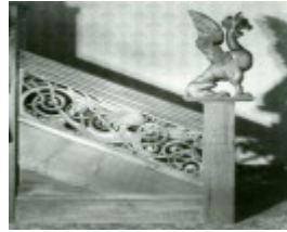
B5468 Dacre Staircase Detail
