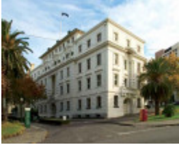
B2692 Commonwealth Offices
