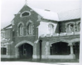
B2715 Clarke Building Trinity College Parkville
