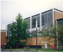
B6318 Beaurepaire Building
