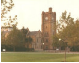
B6489 Old Arts Building
