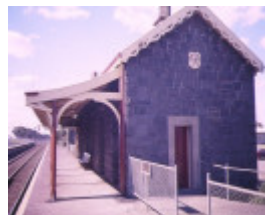
little river station & goods yard school road little river platform side view aug1997
