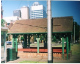
B7050 Tram Shelter
