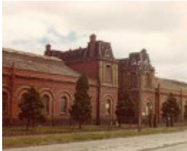
B3704 Pumping Station
