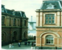
B3704 Spotswood Pumping Station
