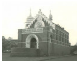
B4899 Court House Flemington
