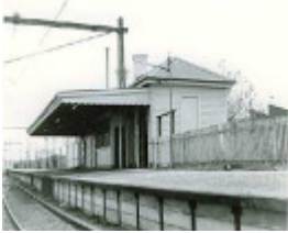
B4023 Williamstown Pier Station
