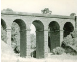
B1787 Railway Viaduct, Sunbury
