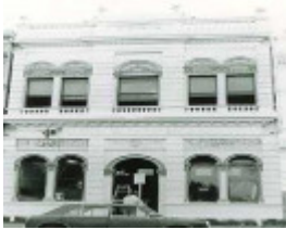
B2505 Advertiser Building Williamstown
