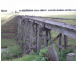
B3033 Bolinda Railway Viaduct 2011
