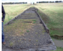
B3033 Bolinda Railway Viaduct deck 2011
