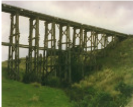
B3033 Bolinda Creek Railway Viaduct
