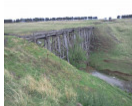
B3033 Bolinda Railway Viaduct 2011
