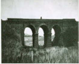
B3894 Railway Viaduct
