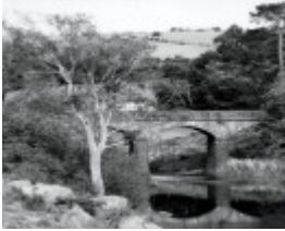
B0910 Bluestone Bridge
