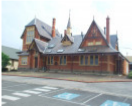
PRIMARY SCHOOL NO. 2120 SOHE 2008
