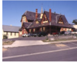
1 former primary school number 2120 long gully front view
