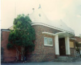
B6471 Old Shire Hall
